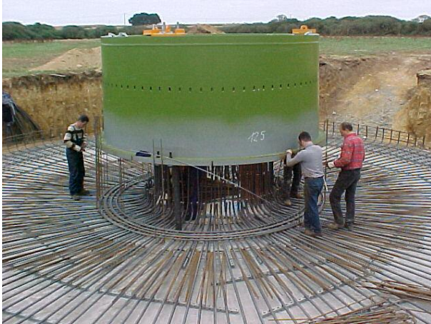
Construction of the foundations
