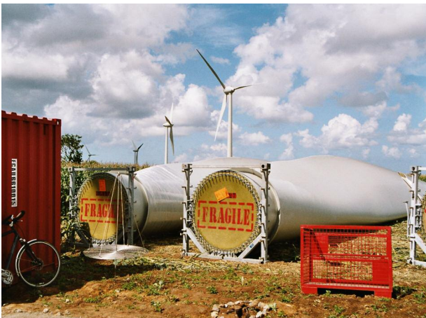
Preparation for the final assembly of the blades
