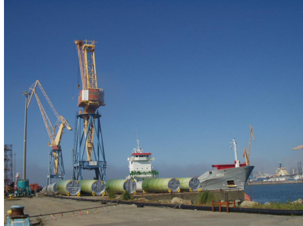
Delivery of the turbine towers at the harbour of Brest
